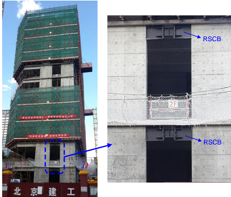
(a) Photograph of prototype building under construction
